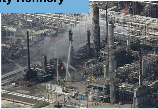
Texas City Refinery
